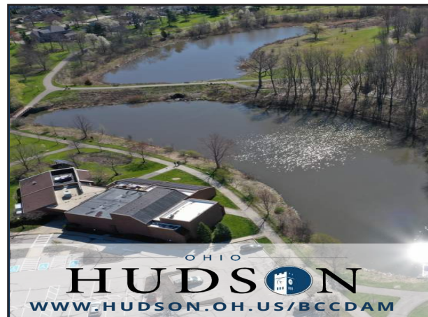
In Hudson, both dams were out of ODN compliance. NEORS reconstructed the Lower Lake Dam in order to safely pass the required design flood flows without over-topping the embankment and construct a new emergency spillway. The Upper Lake Dam's emergency spillway was built. Valve 4: Both Lakes: Upgrade existing electronic valve systems that are opened ahead of storm events. The cost of the project was $1.7M.
